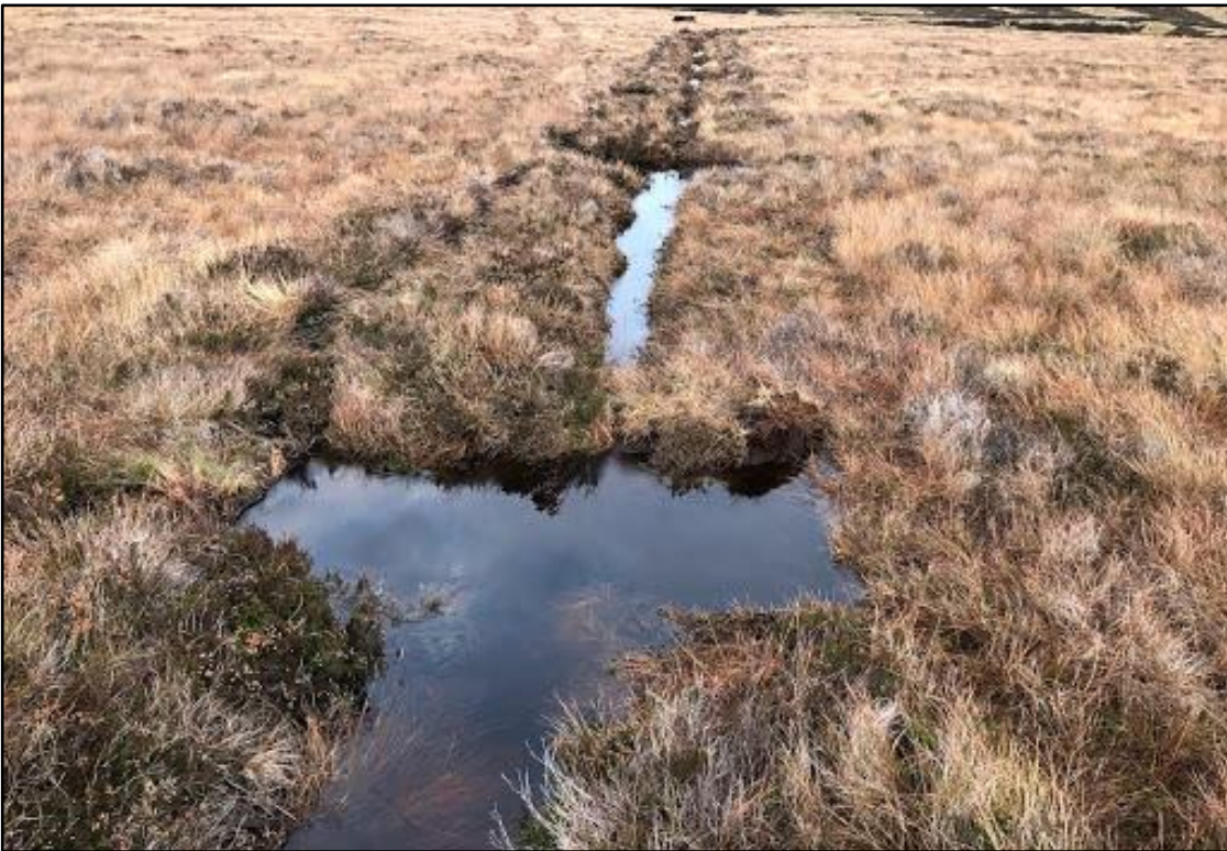
Plate 2.3 Example of peat dams to be used for on-site forestry drain blocking. This will re-establish and maintain a hydrological regime for the required peatland rehabilitation.
